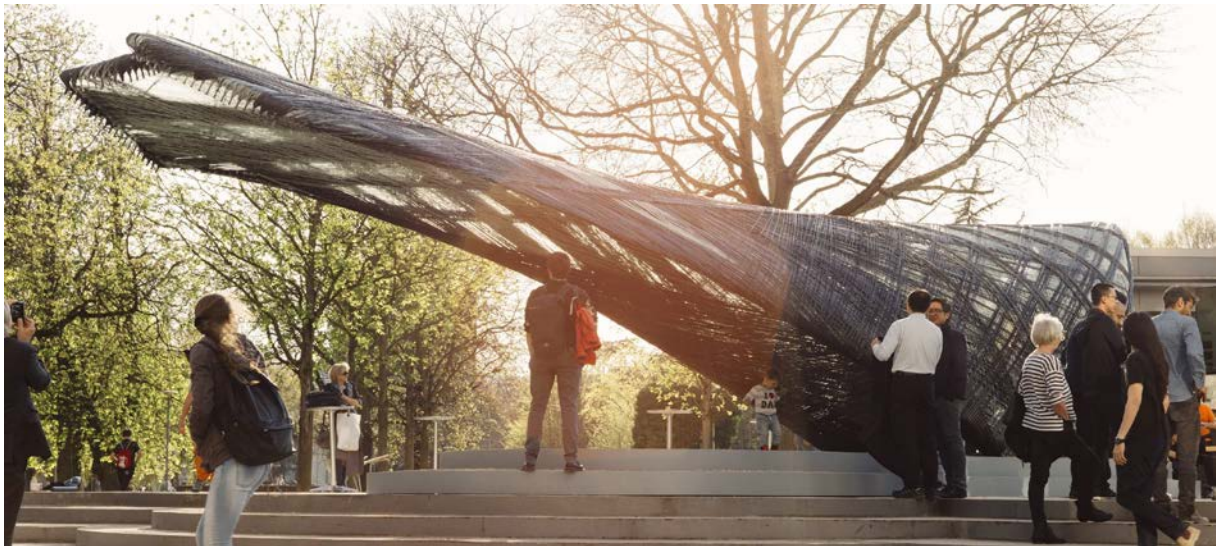
Figure 1: ICD/ITKE research pavilion 2016/2017 at the opening event in March 2017 in Stuttgart
