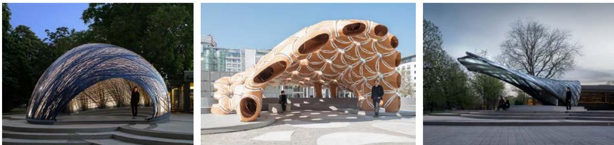
Figure 4: (left to right) ICD/ITKE Research Pavilion (RP) 2014/2015: An FRP-reinforced pneumatic. ICD/ITKE RP 2015/2016: A robotically-sewn wooden-veneer double layered shell. ICD/ITKE RP 2016/2017: A robotically woven FRP cantilever.
